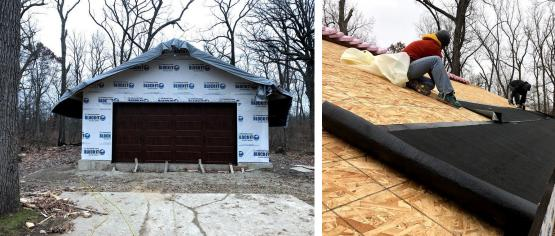
In December we installed the garage door and the last of the fascias, and started the roofing.
