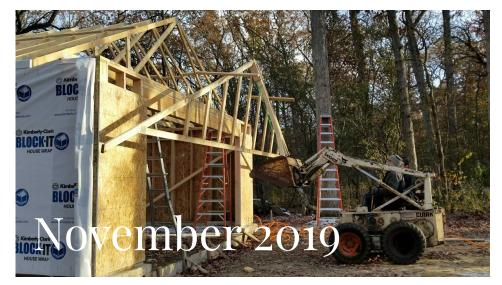
In November we finished the rest of the wall sheathing, installed the final truss, and started sheathing the roof. And it snowed, again, sigh.
