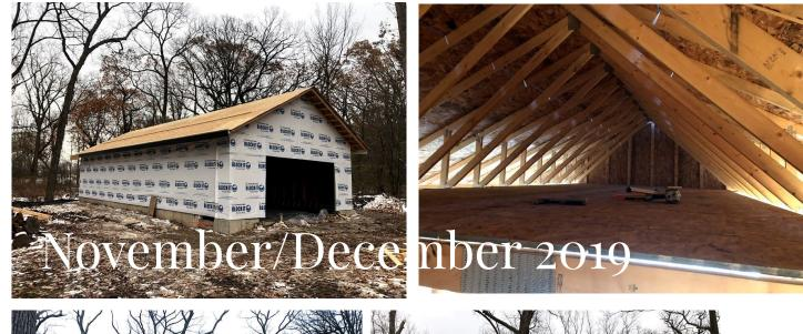
We finished sheathing the roof, built the "clubhouse," and installed lateral bracing.
