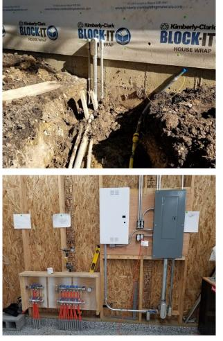
In July we had a trench dug, then worked with an electrician to pull power from the house to Dragonstone. We also installed a gas line for the radiant heating.
