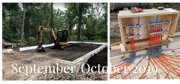
The contractors poured the footings and foundation wall in September, and we installed radiant heating tubes in October and started getting some framing up. The contractors came back and poured over the tubes.
