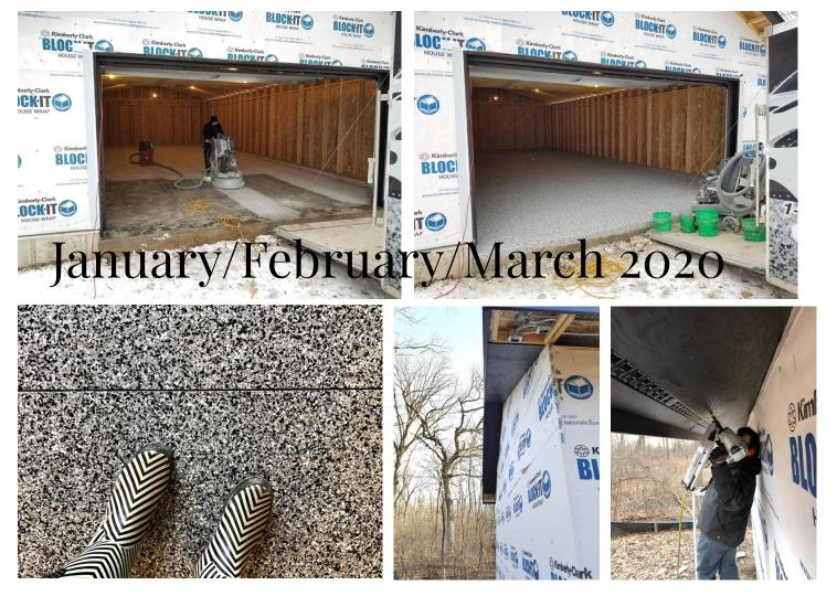
In January we had the floor polyurea coated to protect the concrete. In February we installed exterior conduit. In March, we installed the soffits.
